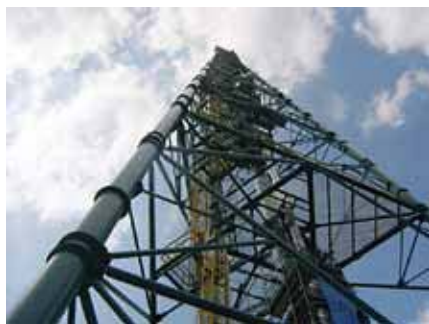
Galvanized steel structures
